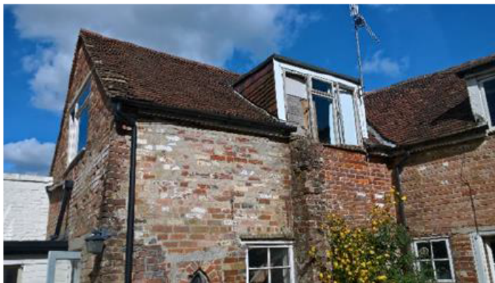
Photograph of the existing building
