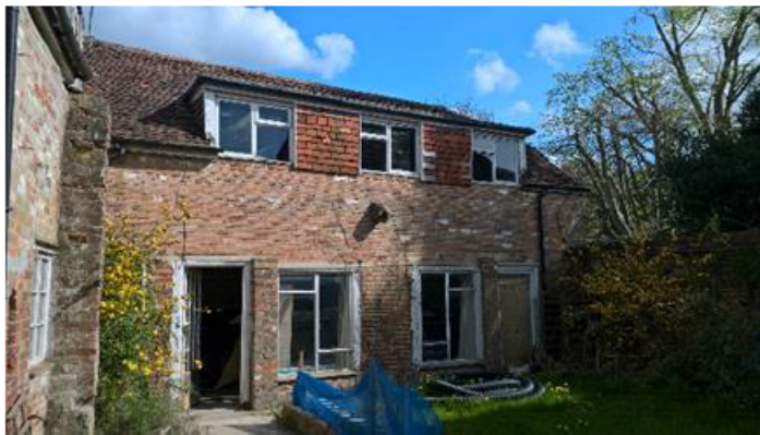
Photograph of the existing building
